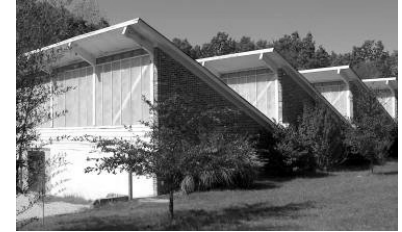
The Solar School
