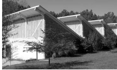
The Solar School
